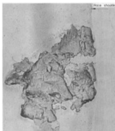
FIG. 3 MULTIPLE SPALL NEAR A RACE SHOULDER
